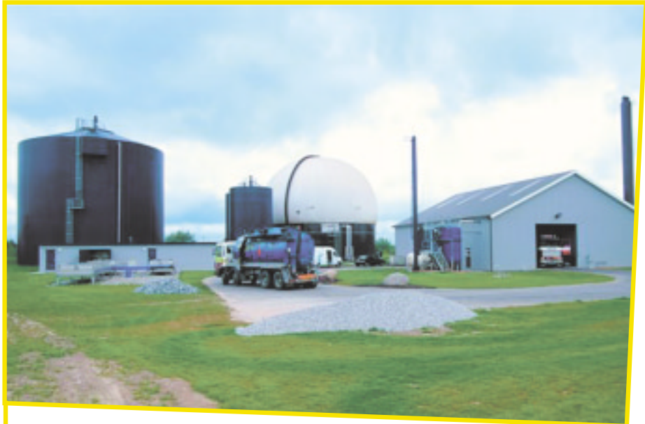
Bio-gas Plant in Denmark
