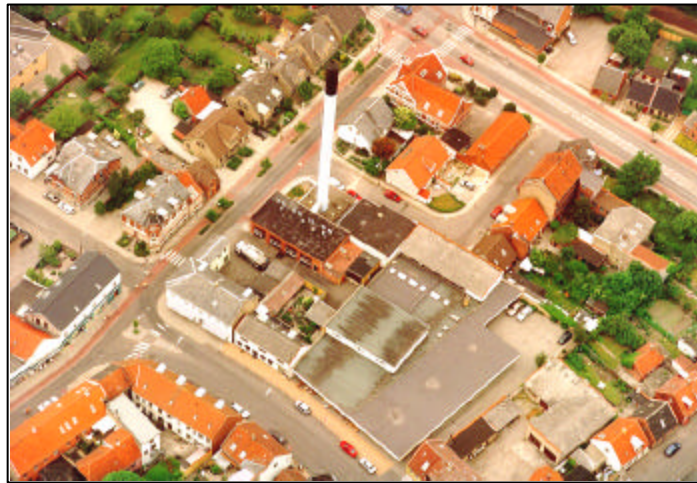
The older plant in the city centre
