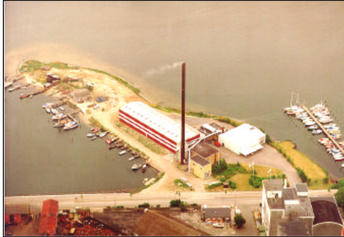
The newer plant.
